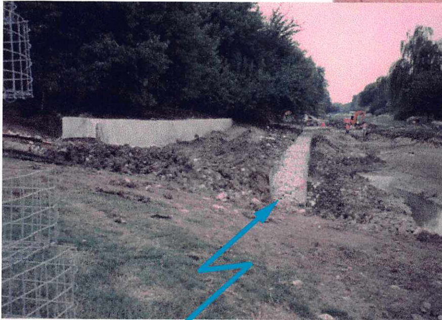
Lake 9 wall under construction.
